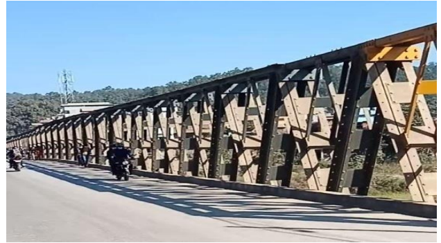
Figure 2 : Girwari bridge-steel bridge
