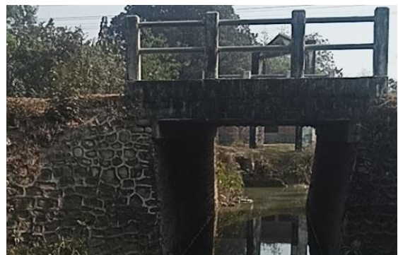
Figure 4 : RCC slab culvert
