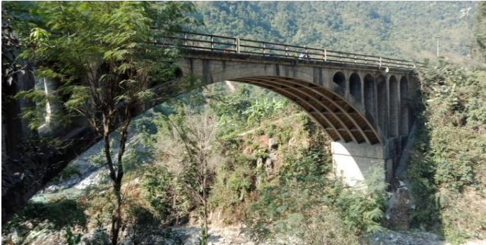
Figure 1 : Khahare khola bridge-arch bridge
