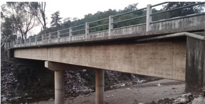
Figure 3 : Martal bridge-RCC T beam
